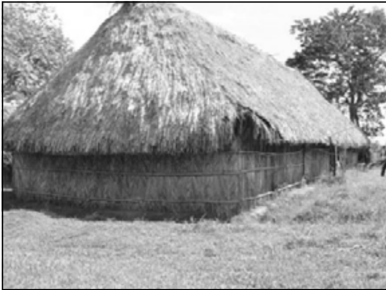
Above The dabuyaba was constructed in 200?? The roof is bay leaf palm and the walls are made from comfra palm ( manicaria saccifera ). The only stands of comfra in Belize are found within the Sarstoon-Temash National Park to the south and west of Barranco. The temple can hold up to three hundred people. The Garifuna believe that death is of the flesh only and that the soul lives on. Part of the purpose of ceremonies will be to communicate with ancestral spirits and also for healing.
